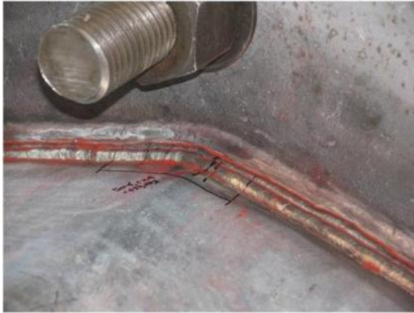
Figure 3.2 Poor Magnetic Particle Test Reading Caused by Geometric Discontinuity
