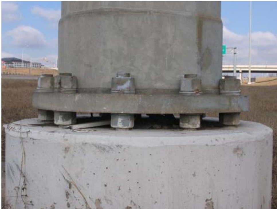
Figure 2.8 Typical High Mast Illumination Pole with External Collar
