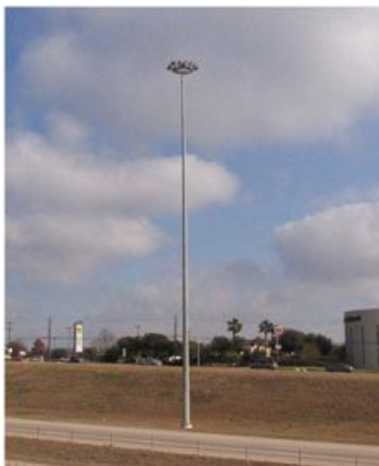
Figure 1.3 Tall Cantilever Design of High Mast Illumination Pole
