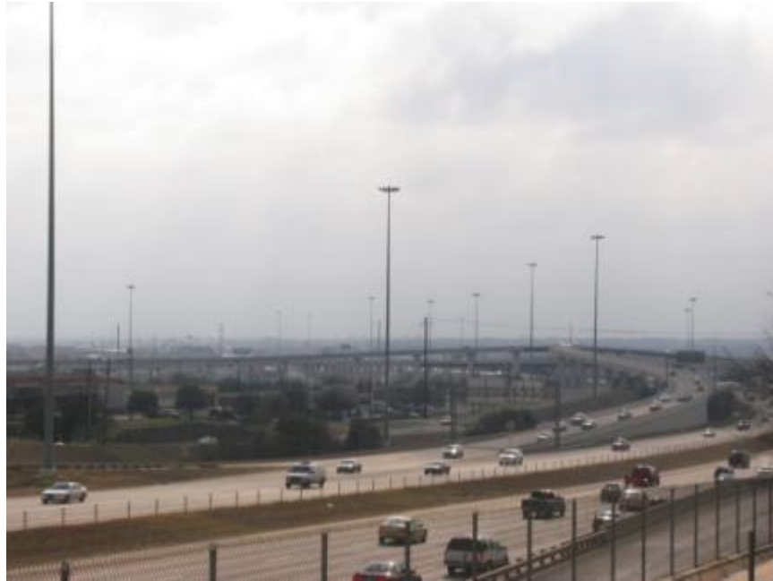
Figure 1.2 Typical High Mast Towers around a Highway Interchange (Rios, 2007)
